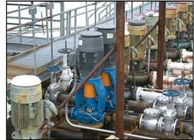
*Goulds vertical in-line Model 3996 process pumps, controlled by PumpSmart, help provide the correct blend of ethanol and gasoline at Motiva distribution terminals in the Northeast USA.*
